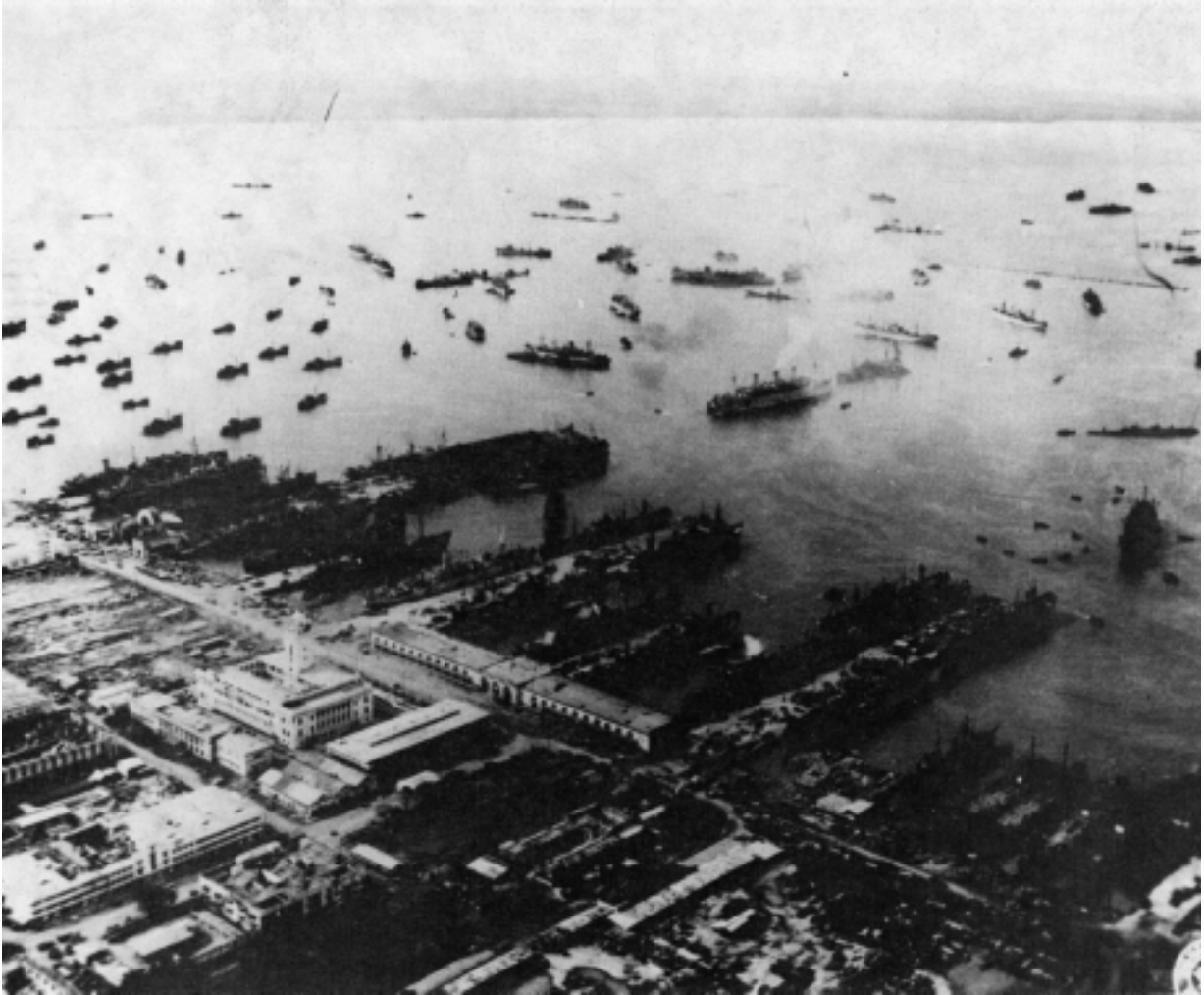
Port of Manila. Under Trudeau's Base X command, Manila handled 20,000 tons of cargo daily in preparation for the invasion of Japan.
